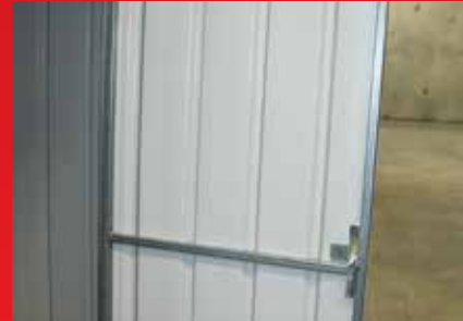
Upgrade to Steel Frame Door and Opening
